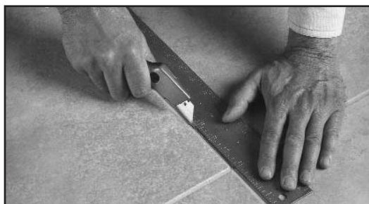
Fig. 27 - Cut along the center of the grout line after heating it.
