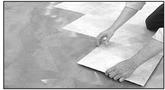
Fig. 14 - Install ungrouted floors following a stair-step pattern.
