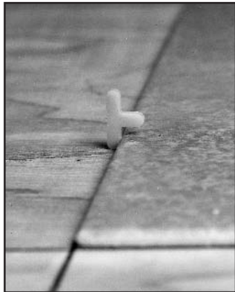
Fig. 11 - Use spacers with one leg removed.
