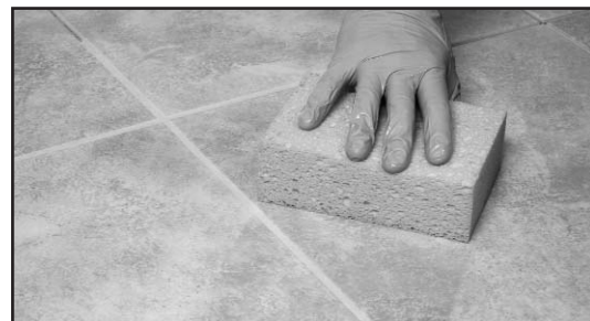
Fig. 22 - Wipe diagonally across the joints to remove excess water.
