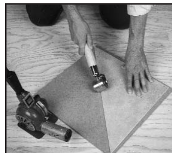
Fig. 18 - Roll the cut edge to form a slight radius.
